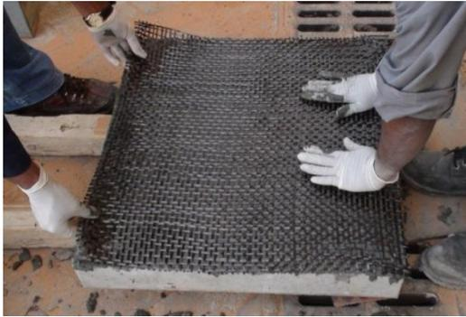
(e) Pressing on fabric for mortar penetration
