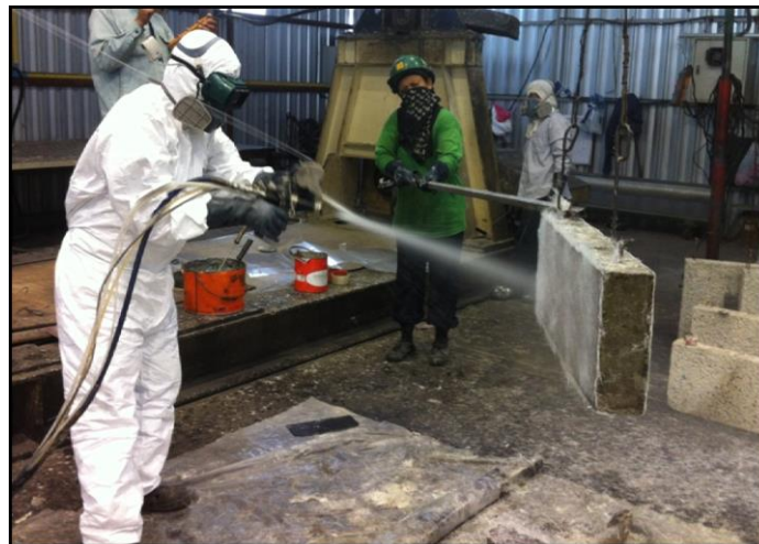
Figure 4: Spraying process of RC deep beams.
