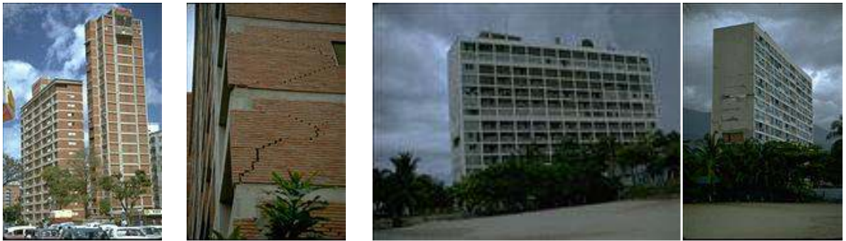
(a) Petunia buildings, with one line of defense (masonry walls) in the short and slender direction. Large plan aspect ratio
