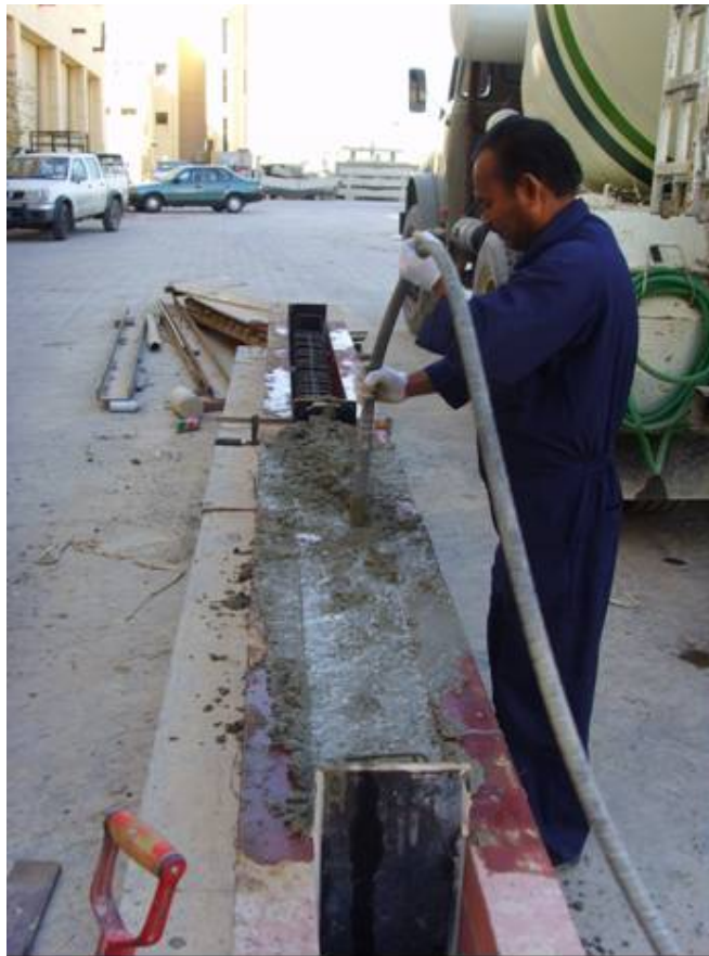
Figure 9 Casting of RC beams using ready mix concrete.
