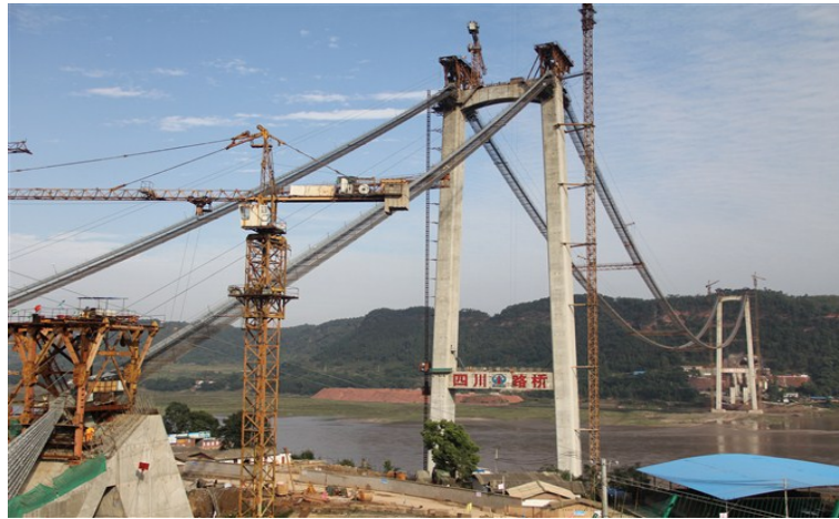
Figure 5: Layout of Nanxi Yangtze Bridge during construction.
