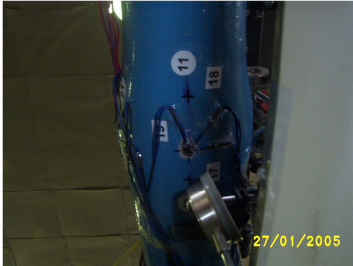
Figure 7 Failure Mode F: local buckling of the chord face.
