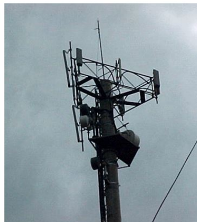
(a) Photographs of the tower
