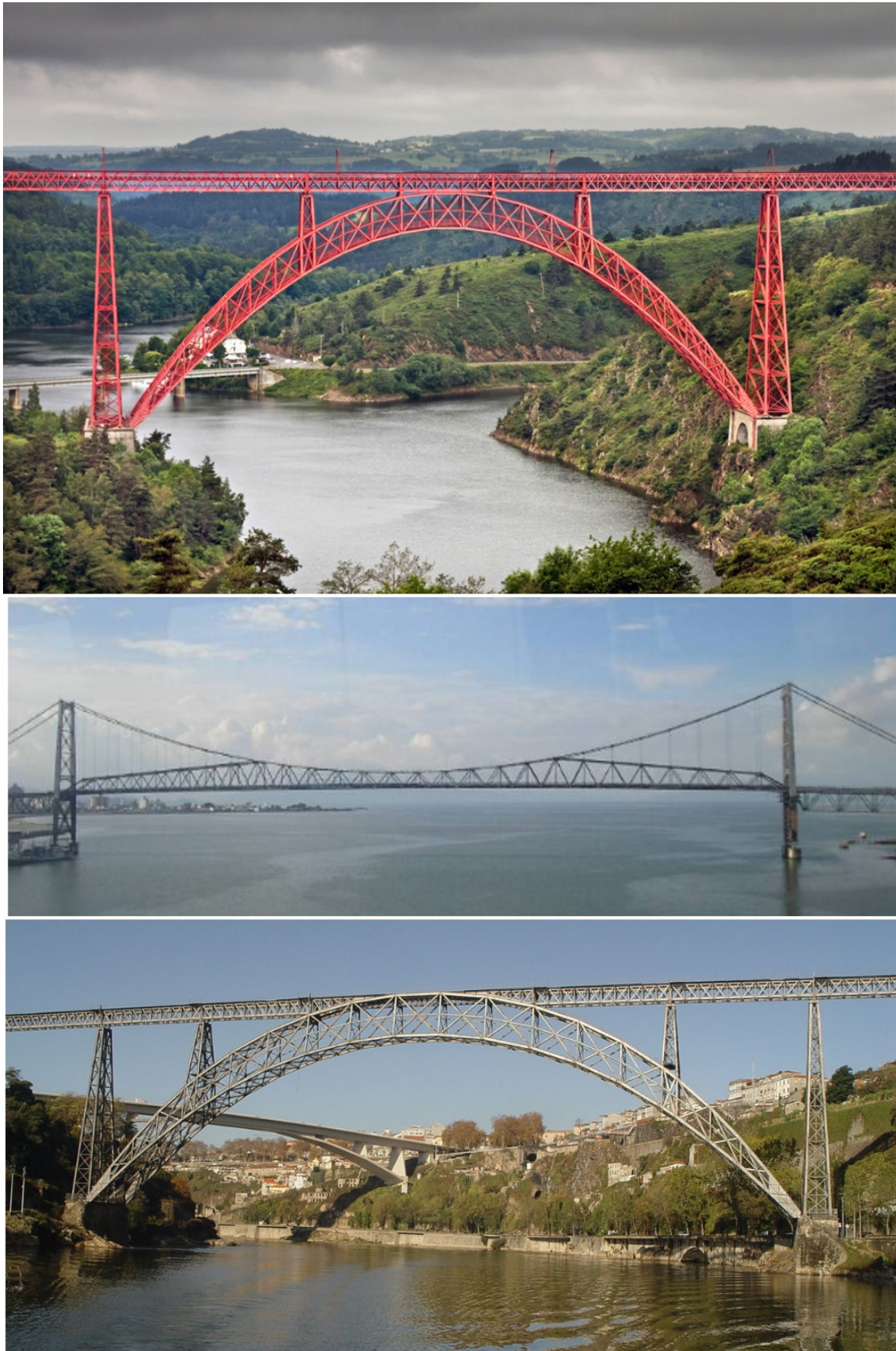
Figure 3: The Garabit Viaduct (G. Eiffel), Ponte Hercílio Luz (Robinson and Steinman), Ponte Maria Pia (G. Eiffel and T. Seyrig).
