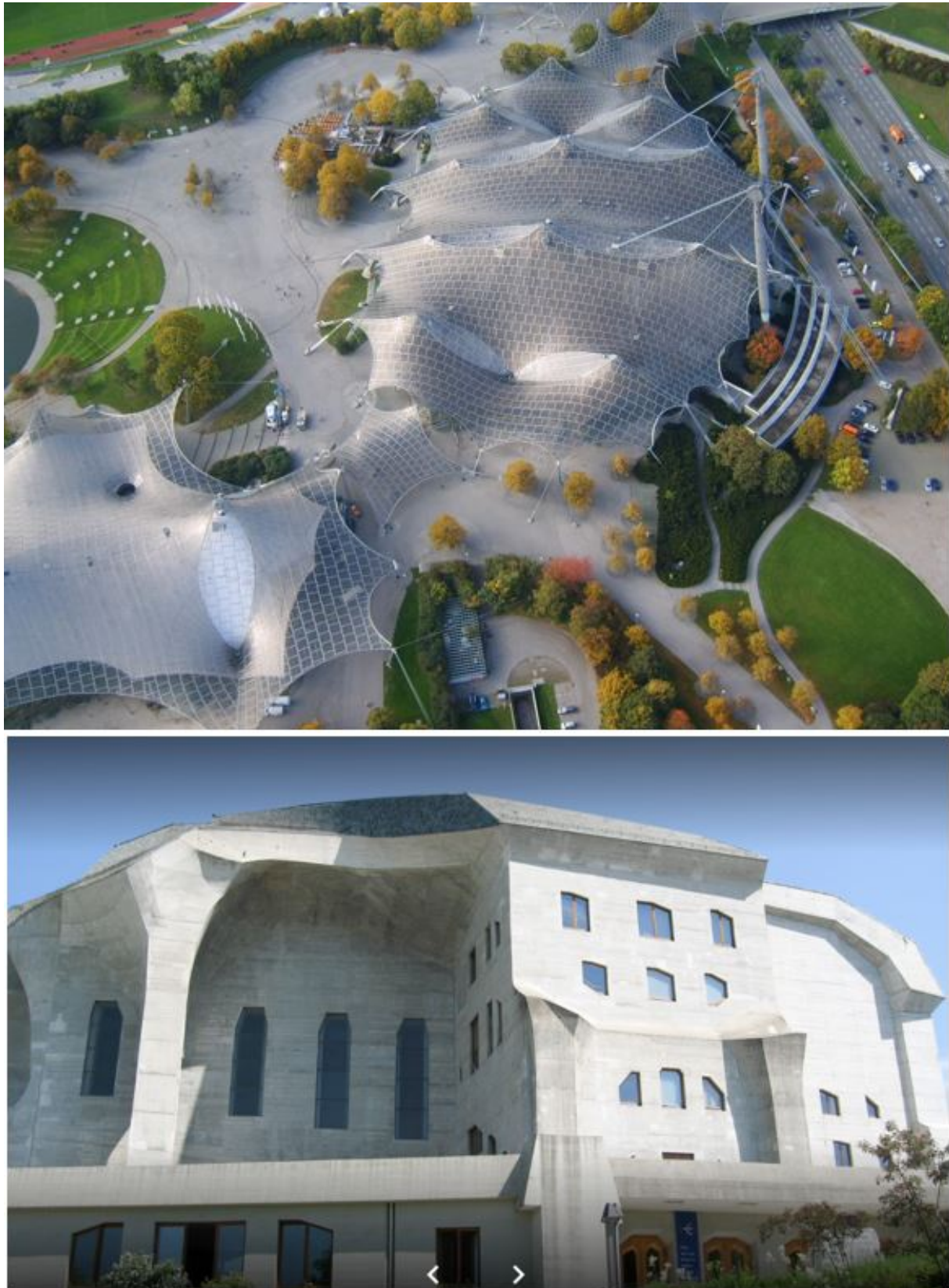
Figure 8: The Olympia Park and the Goetheum as examples of 3D tensile and reinforced concrete structures.
