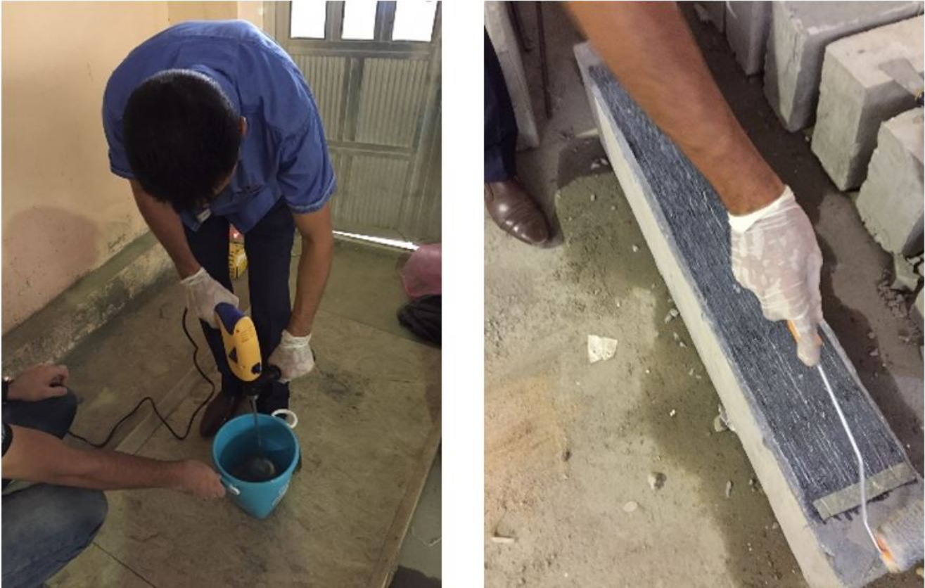
Figure 2. Mixing and application of Epoxy Resin
