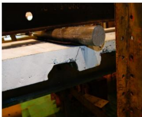
a) Transverse crack underneath point load
