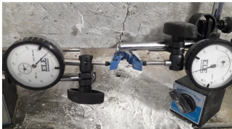
Figure 5. Micro-crack opening displacement measured using mechanical dial gauges
