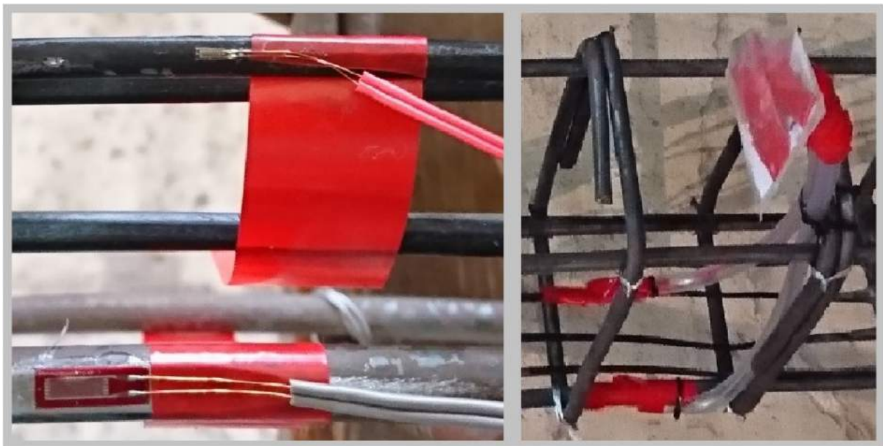
Figure 3. Fixing, isolation, and protection of the strain gauges.
