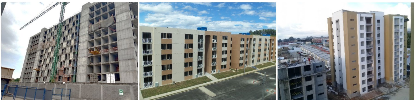
Figure 1. Reinforced concrete thin walls buildings.
