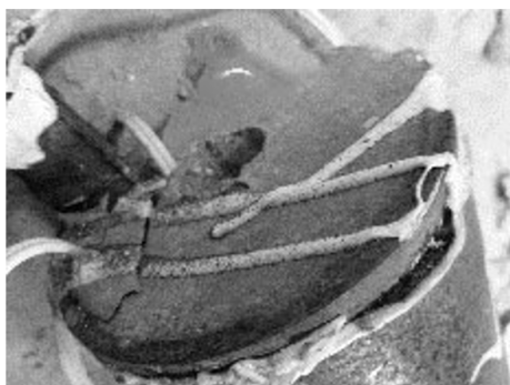
(a) Bar failure of fixed end
