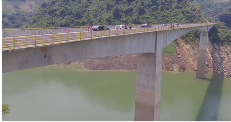
Figure 1. View of the Pujamanes Bridge
