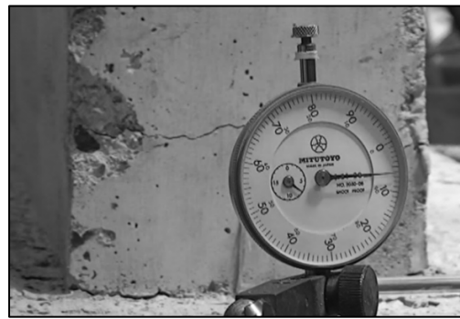
Figure 13 Cracking at the bottom.
