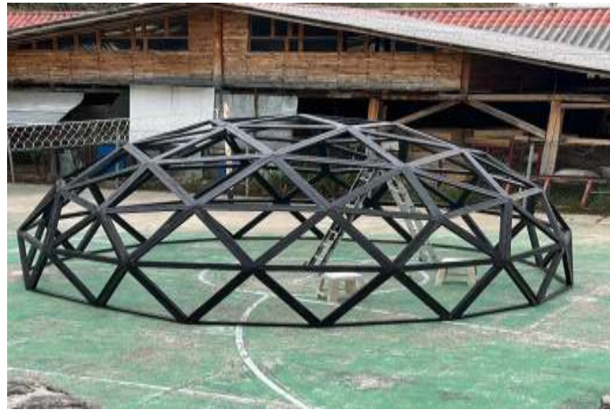
Figure 18 Geodesic dome with recycled polypropylene plastic elements.
