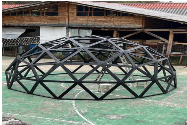
Figure 18 Geodesic dome with recycled polypropylene plastic elements.
