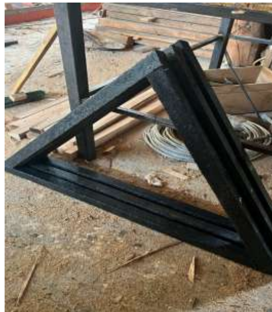
Figure 16 Connection of Elements to Form the Triangles of the Frequency 3 Dome.
