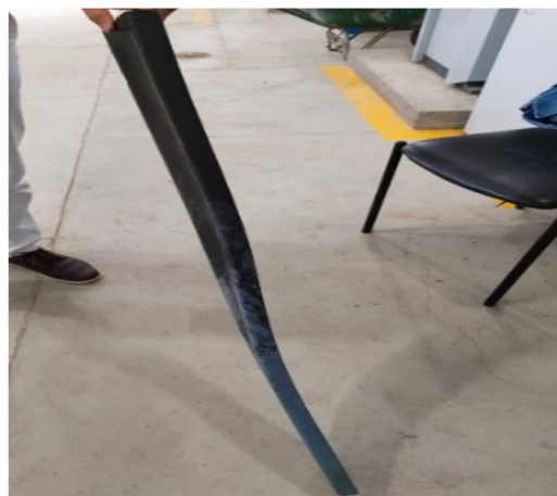
Figure 9 Example of Lateral Torsional Buckling in a Tested Structural Element
