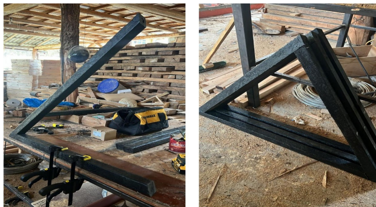
Figure 16 Connection of Elements to Form the Triangles of the Frequency 3 Dome.
