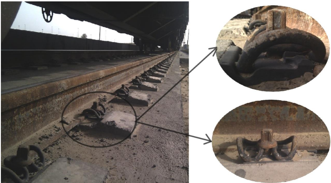
Figure 1: Vossloh spring clips-type SKL14
